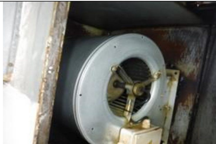
6.Fan Unit after
