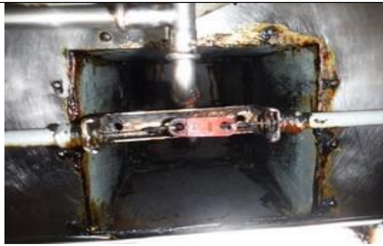
2. Ductwork 1M from canopy after
