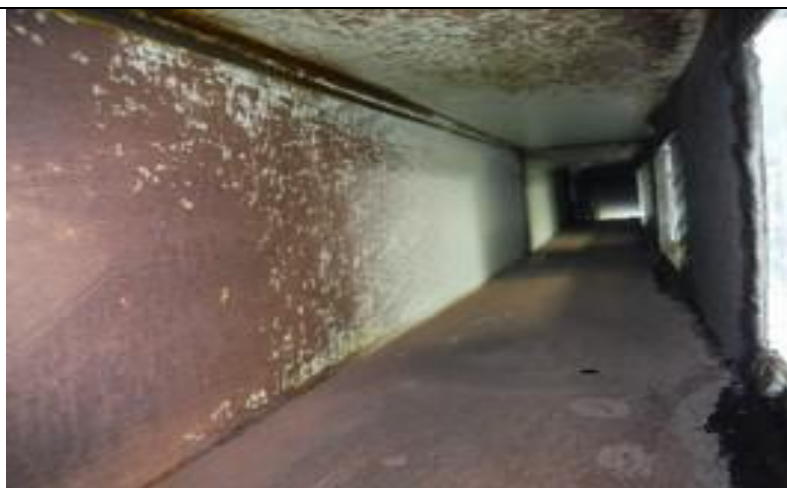
3. Ductwork 3M from canopy before
