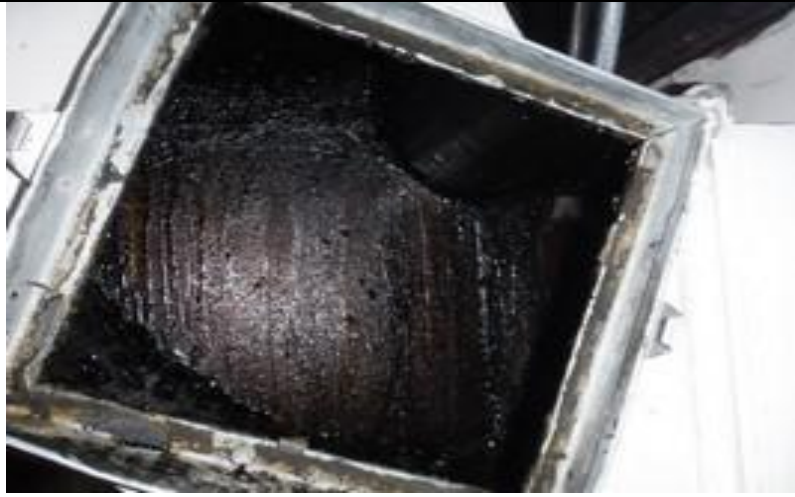
5. Ductwork Upstream of Fan before
