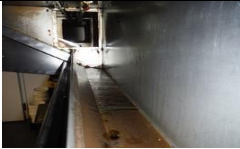
1.Canopy plenum (Basement Extract)before
