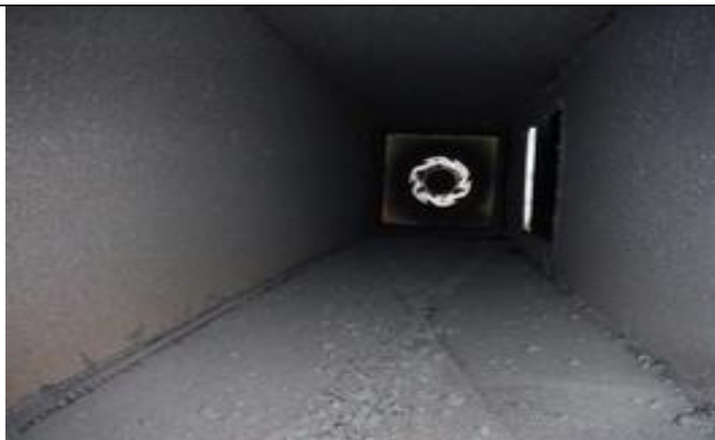
5.Ductwork Upstream of Fan before
