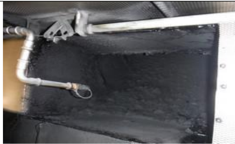
2. Ductwork 1M from canopy before
