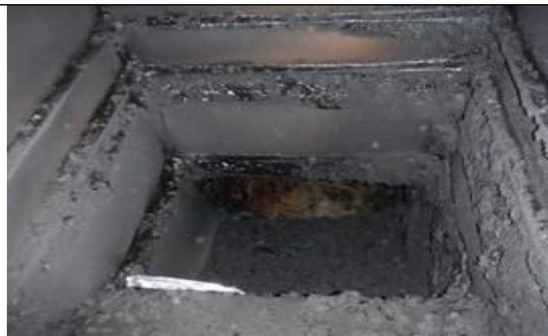
3. Ductwork 3M from canopy before
