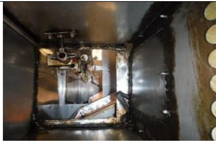
2.Ductwork 1M from canopy after
