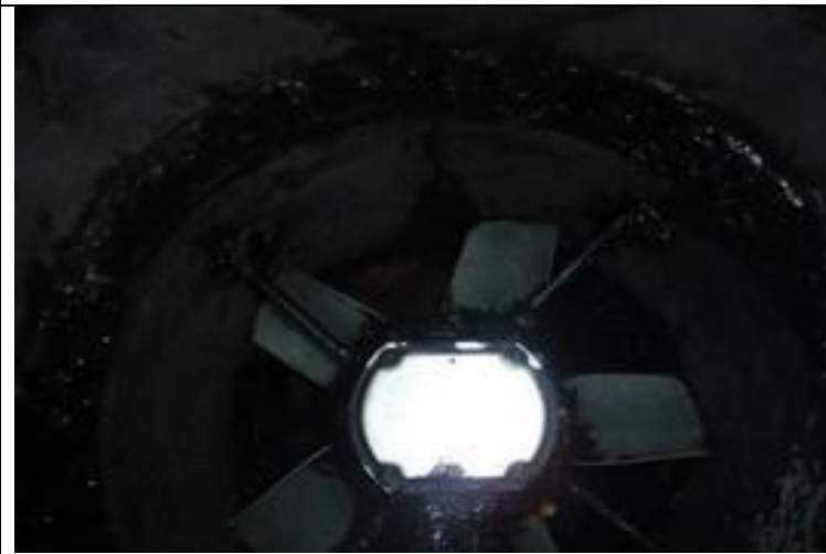
7. Ductwork Downstream of Fan after
