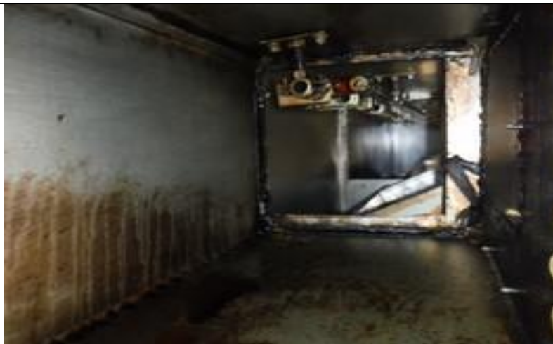
2. Ductwork 1M from canopy before
