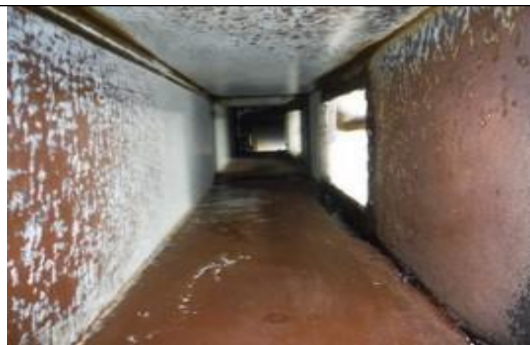
3. Ductwork 3M from canopy after
