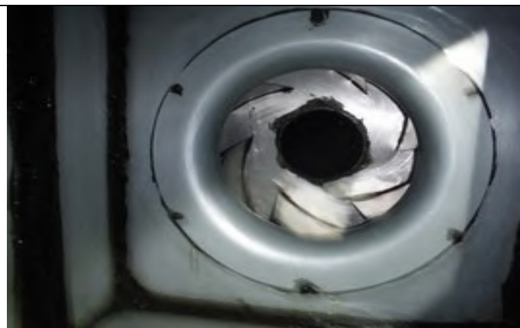
6. Fan Intake after
