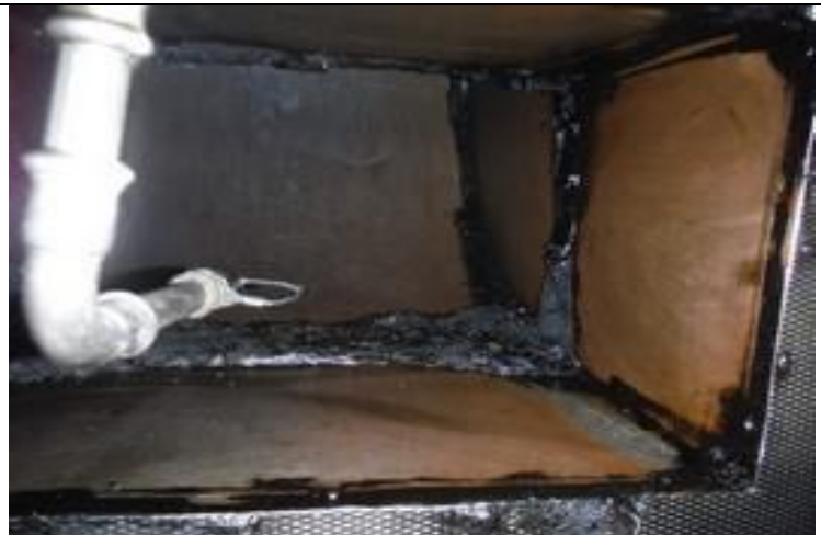
2. Ductwork 1M from canopy after
