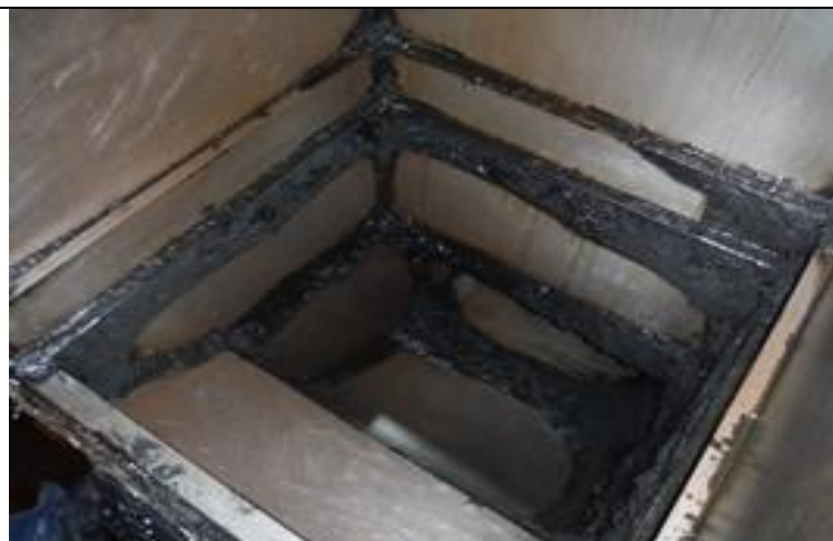
3. Ductwork 3M from canopy after
