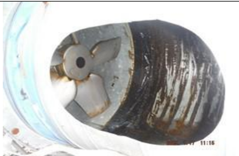
5. Duct upstream of fan after
