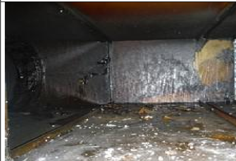
Filter box before
