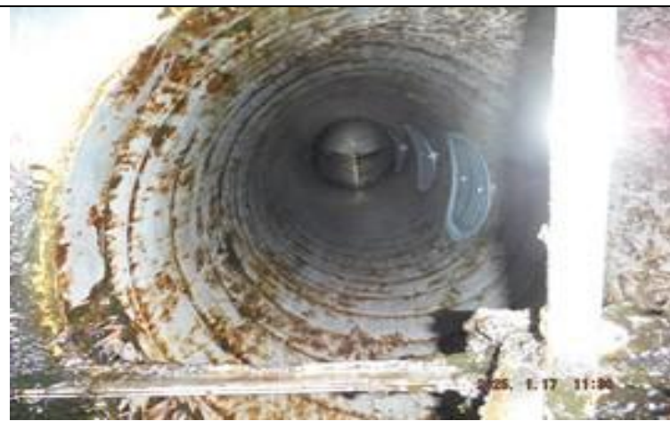
2. Ductwork 1M from canopy after
