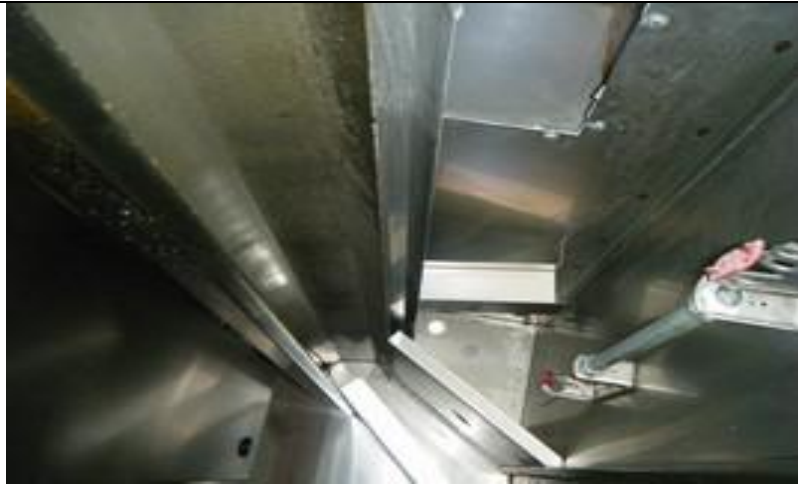
1 Canopy plenum before
