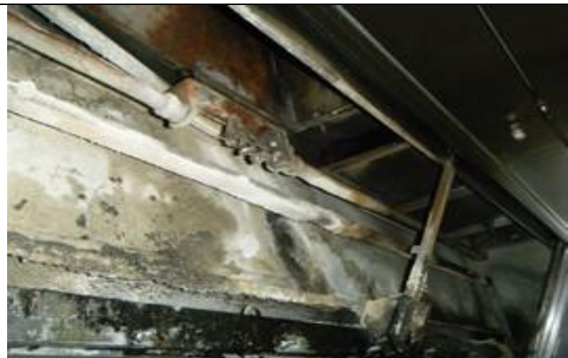
1. Canopy plenum 3 before
