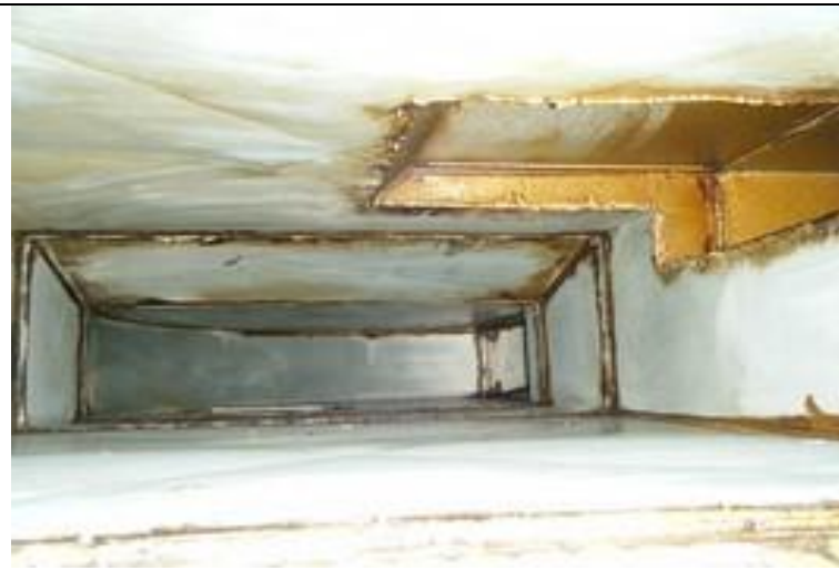
3 Ductwork 3M from canopy after
