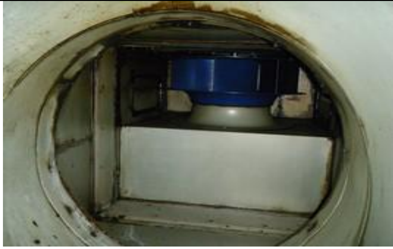
6.Fan Unit before
