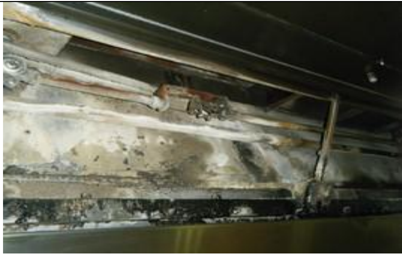
2 Ductwork 1M from Canopy before
