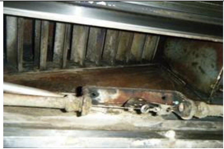
2. Ductwork 1M from Canopy after
