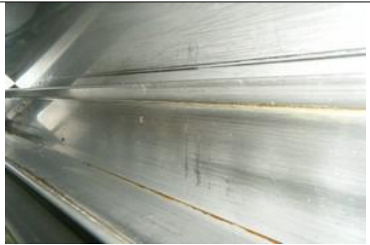
1.Canopy plenum 2, after
