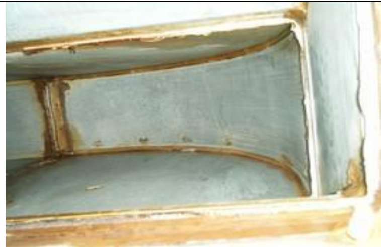
2. Ductwork 1M from Canopy 2 after
