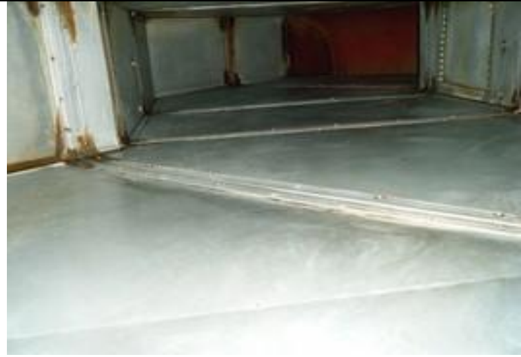
5. Ductwork Upstream of fan ( roof area) after
