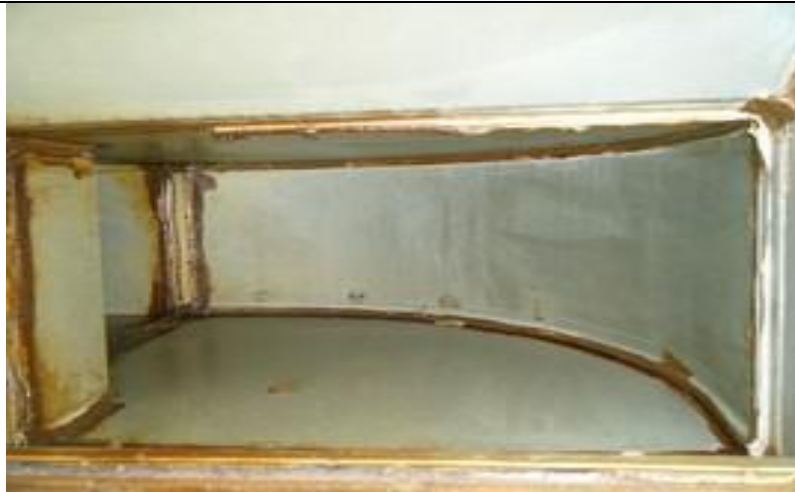
2. Ductwork 1M from Canopy 2 before
