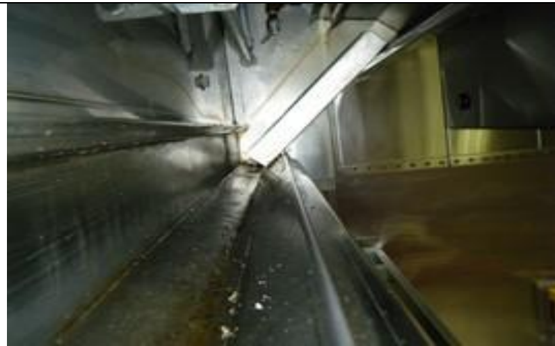
1. Canopy plenum 2, before
