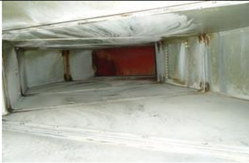
5. Ductwork Upstream of fan ( roof area) before
