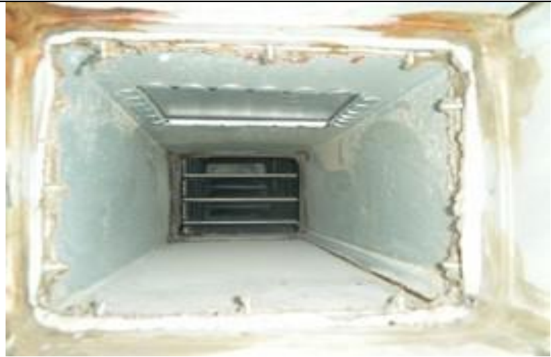
2. Ductwork 3M from Canopy 4 before
