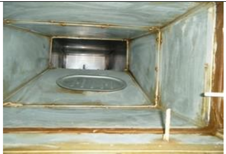
3. Ductwork 3M from canopy after
