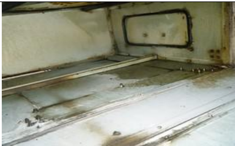
5. Ductwork Upstream of fan ( roof area) before
