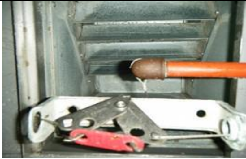
2. Ductwork 1M from Canopy 3 before
