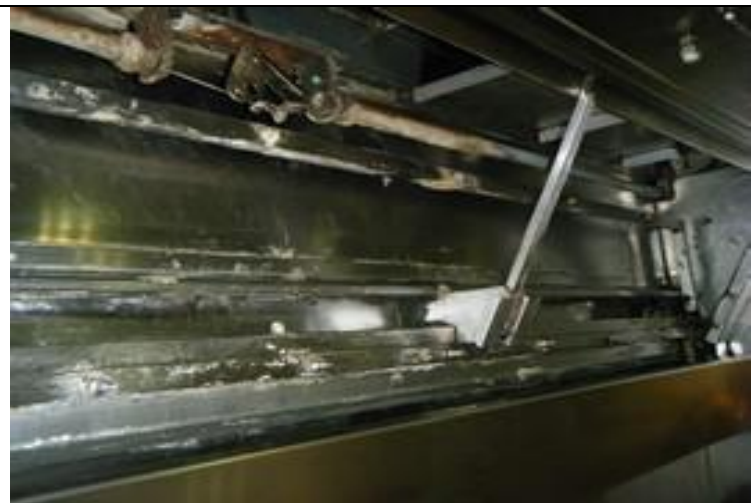
1. Canopy plenum 3 after
