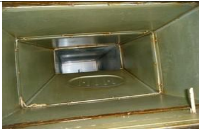
3. Ductwork 3M from canopy before
