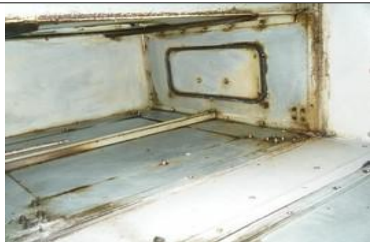
5. Ductwork Upstream of fan ( roof area) after
