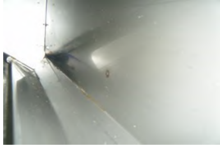
1. Canopy plenum 4 after
