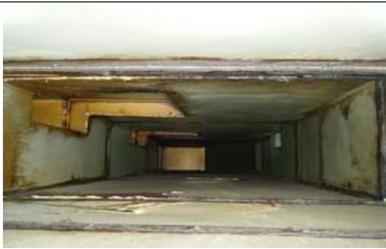
3 Ductwork 3M from canopy before
