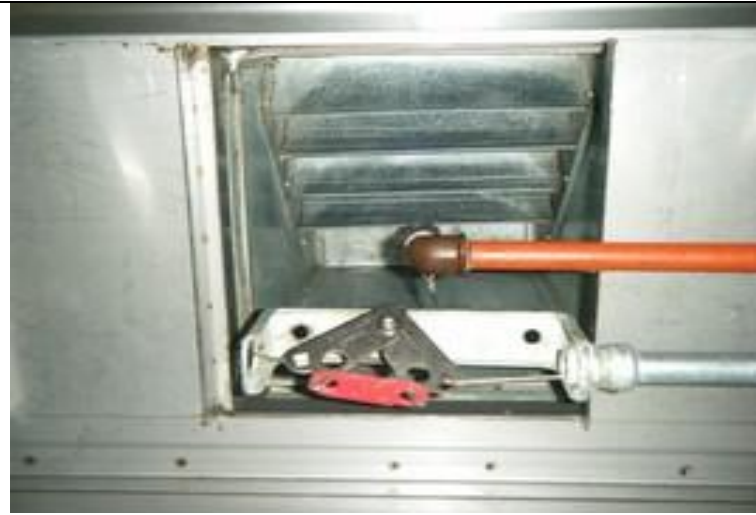
2. Ductwork 1M from Canopy 3 after
