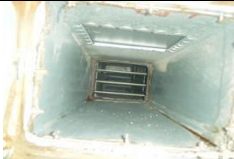
2. Ductwork 3M from Canopy 4 before
