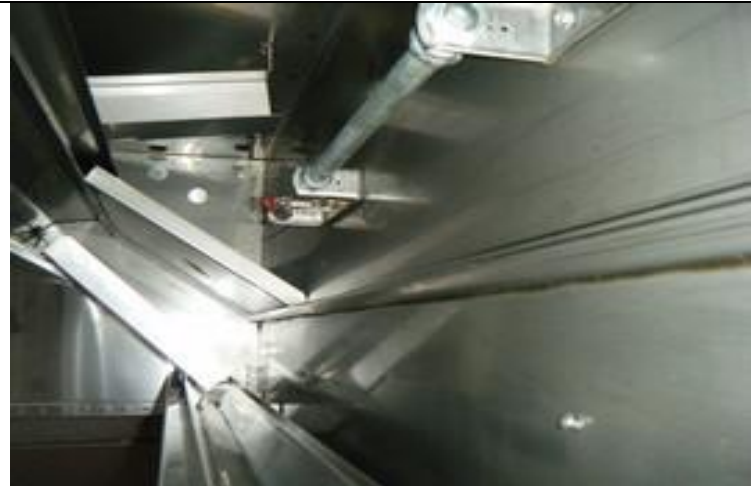
1 Canopy plenum after
