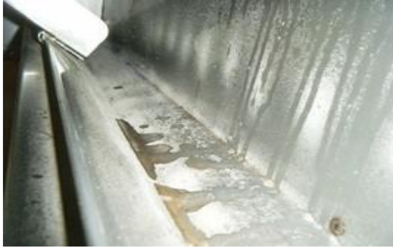
1. Canopy plenum 4 before
